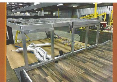
TUBULAR ALUMINUM KNEE WALL CONSTRUCTION, SOME COMPETITION USES 2X2 PIECES OF WOOD.
